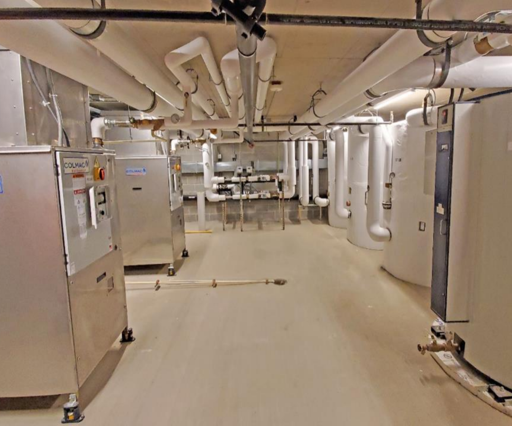
Figure 4. Single-Pass Primary HPWH with Series Temperature Maintenance Tank System (Swing Tank)
