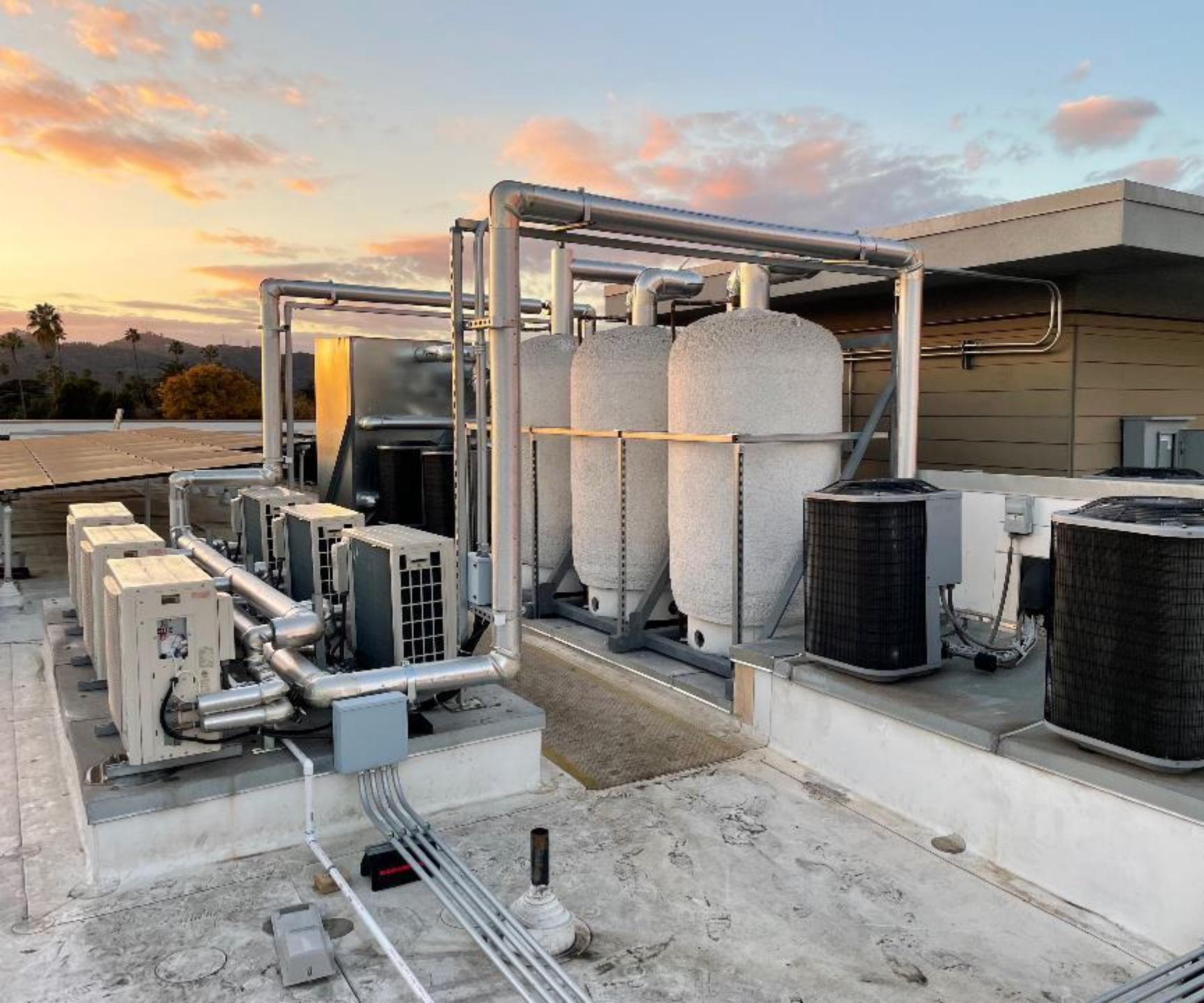
Figure 5. Single-Pass Primary HPWH with Parallel Temperature Maintenance Tank System
