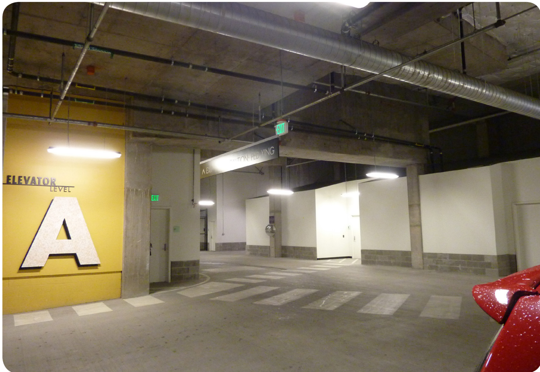
Parking garage with modern linear fluorescent lighting and bright reflective surfaces.
