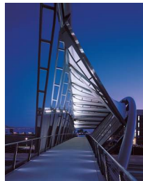
Argen Helix Bridge Johnson Architects
