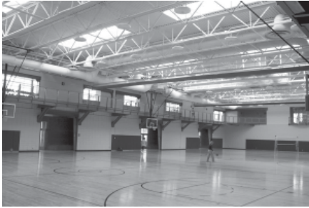
Left: The gymnasiums at the new University of Montana Rec Center integrate daylight and fluorescent lighting into an efficient and visually effective space.
