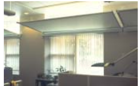
Fig. 2: A lightshelf divides the window into upper daylight glazing and lower view glazing. Visible light transmission may be higher in the upper glazing (to increase daylight) and lower in the view glazing (to minimize glare). Photo credit: Sacramento Municipal Utility District
