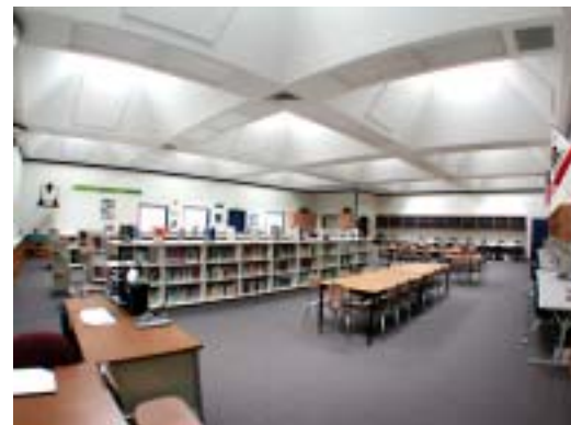
Fig 3: Diffusing skylights spread soft daylight evenly across this library space. Photo credit: SunOptics Skylights
